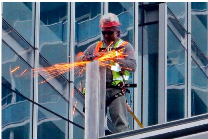
Alan Kotok: Office building construction worker. Flickr CC.
